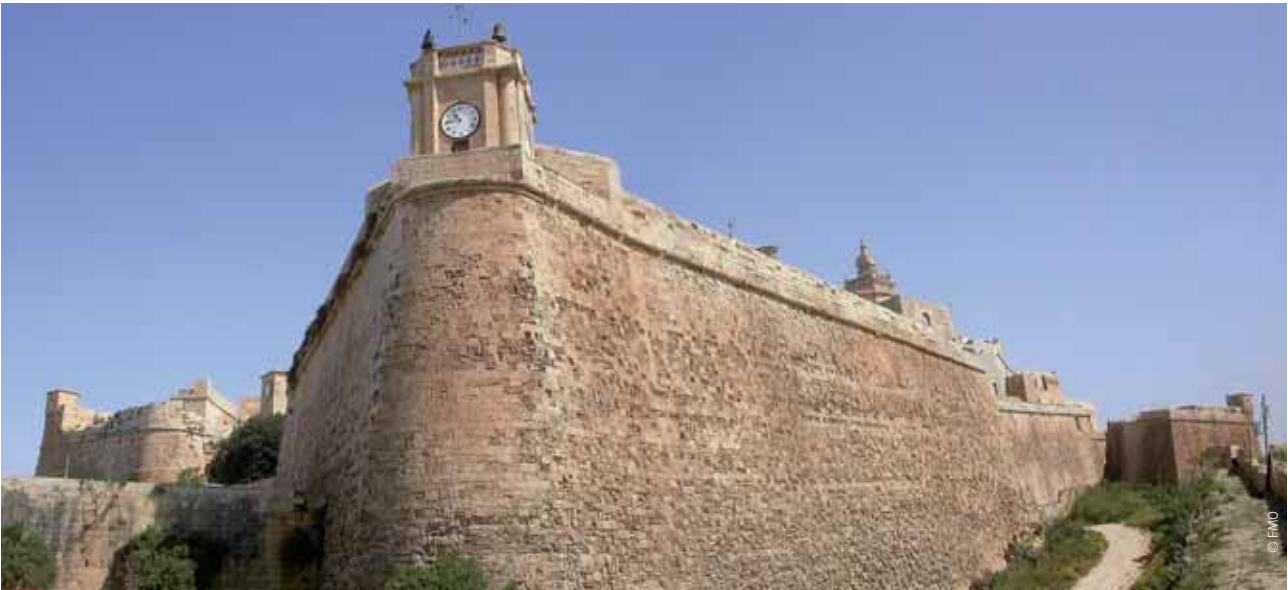
On the small Mediterranean island of Gozo, the EEA Grants have supported the development of a large-scale plan to renovate the Cittadella, the island's main historical site.
