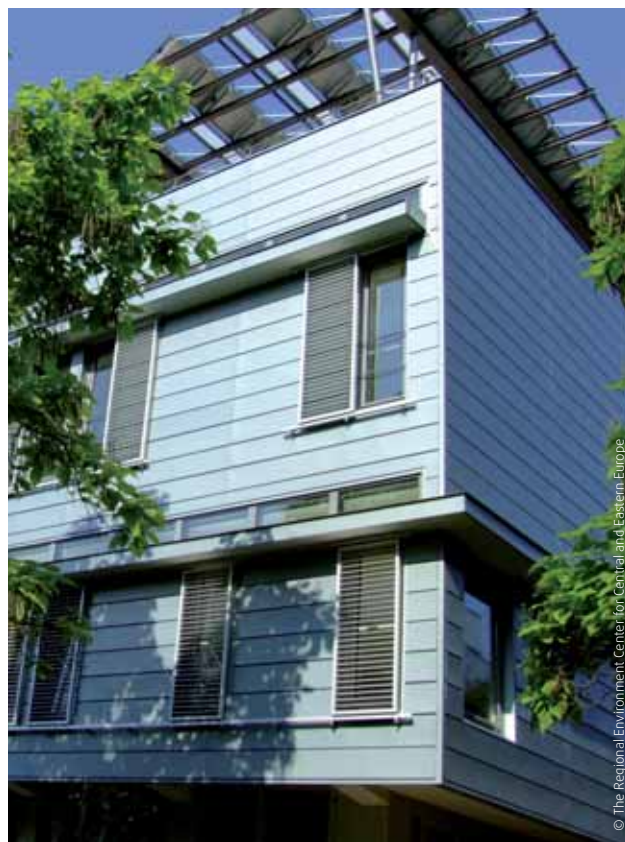
In Hungary, the Regional Environmental Centre has been made into a zero-emissions conference centre.
