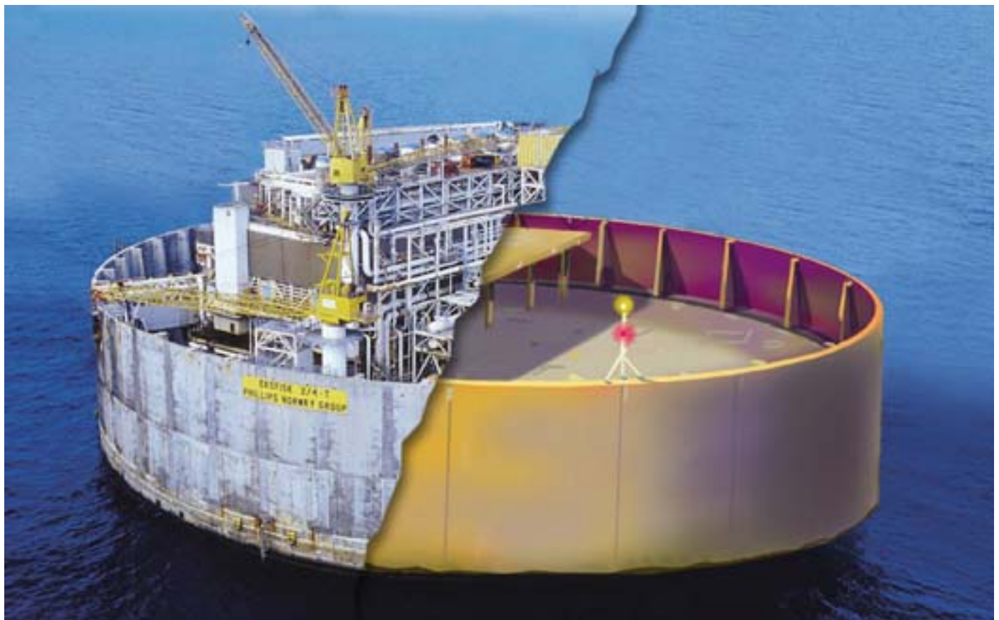
Figure 6.7 Illustration of the Ekofisk tank before and after removal of the topside (Source: ConocoPhillips)
