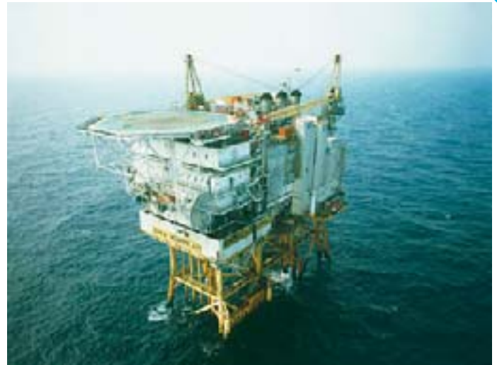
Figure 6.6 The pumping facility 37/4A whose substructure was removed during the summer (Source: ConocoPhillips)
