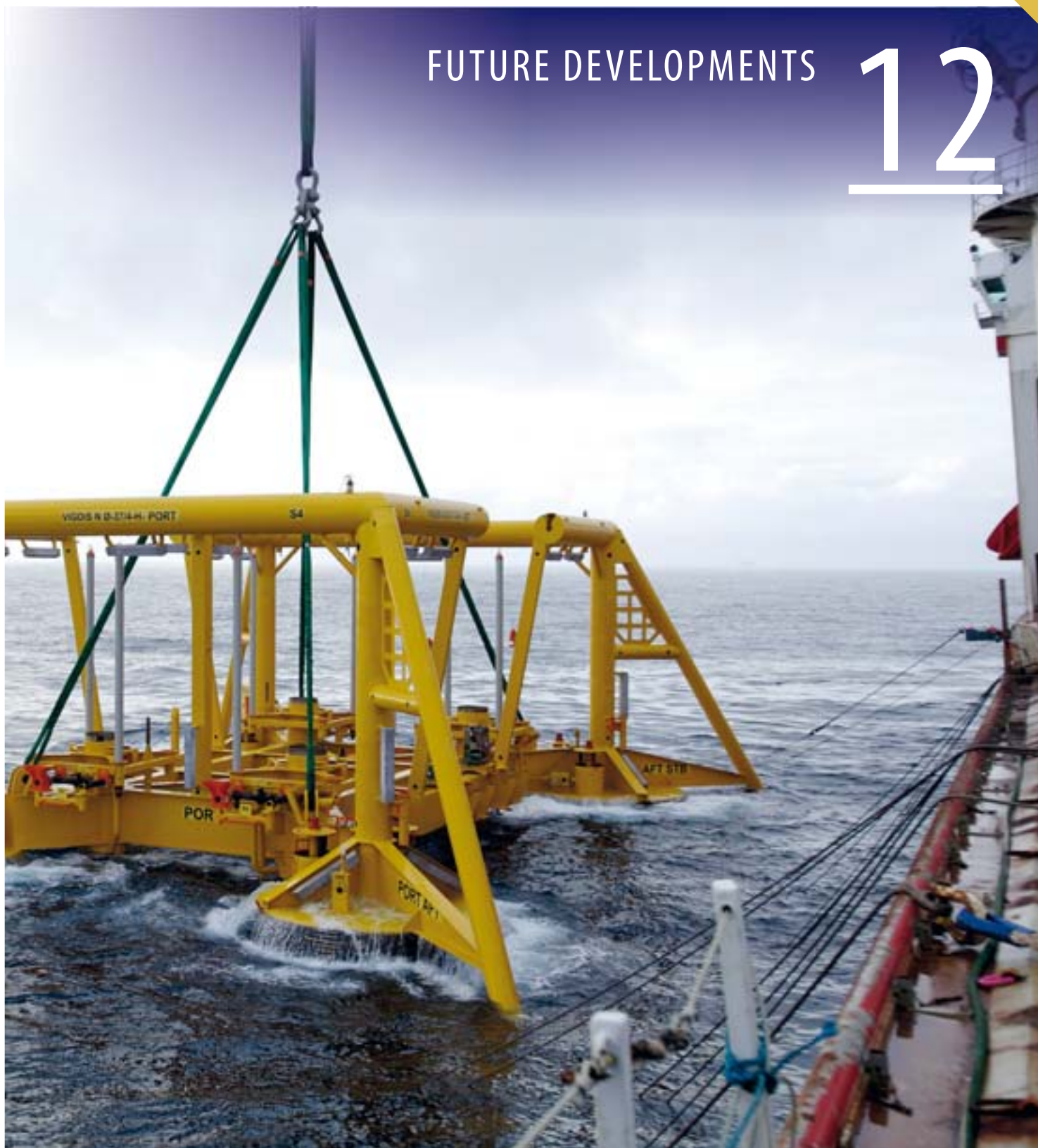
More and more fields are being developed with underwater installations, here showing the installation on Vigdis Øst. (Photo: A. Osmundsen, Statoil)
