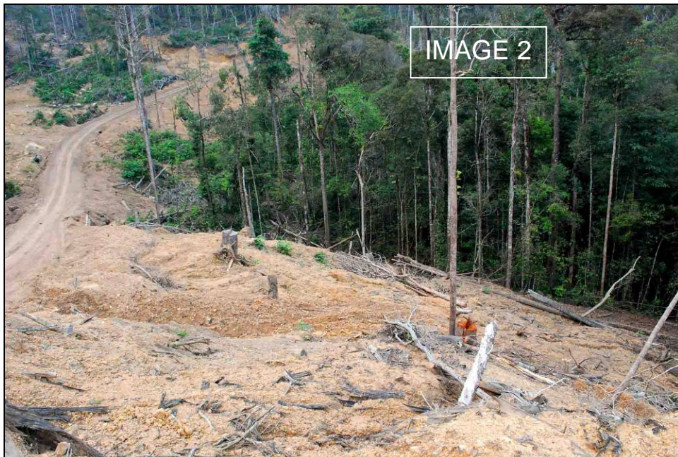
Figure 16: Forest completely cleared for up to 50 metres at the side of the road, in breach of normal limits. See Figure 12 for location.
