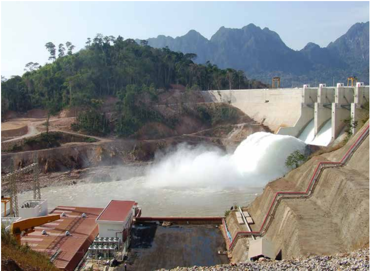
In January 2013 the Lao Theun-Hinboun Power Company (THPC), in which Statkraft owns 20 per cent, opened two new power stations. Like the existing power station, which was completed in 1998, the new stations will be operated and maintained by Statkraft. Overall, the expansion will double the production of renewable energy to 3 TWh per year.
