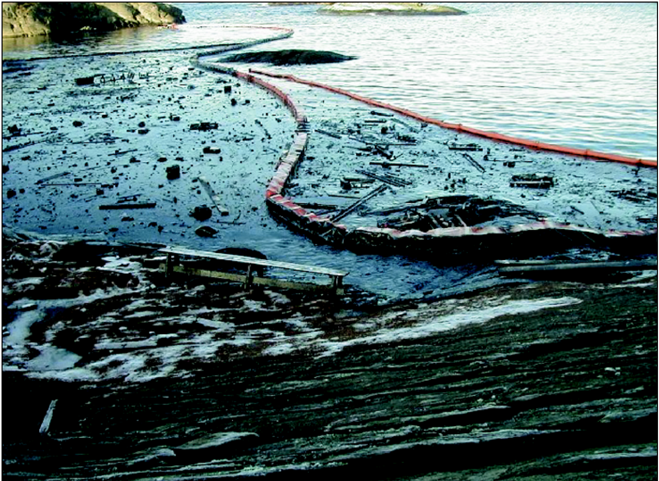
Figure 3.7 The Norwegian Pollution Control Authority's emergency services for combating oil spills at work with bilge pumps in Bleivika near Haugesund after the sinking of the vessel "Green Ålesund" in December 2000.
