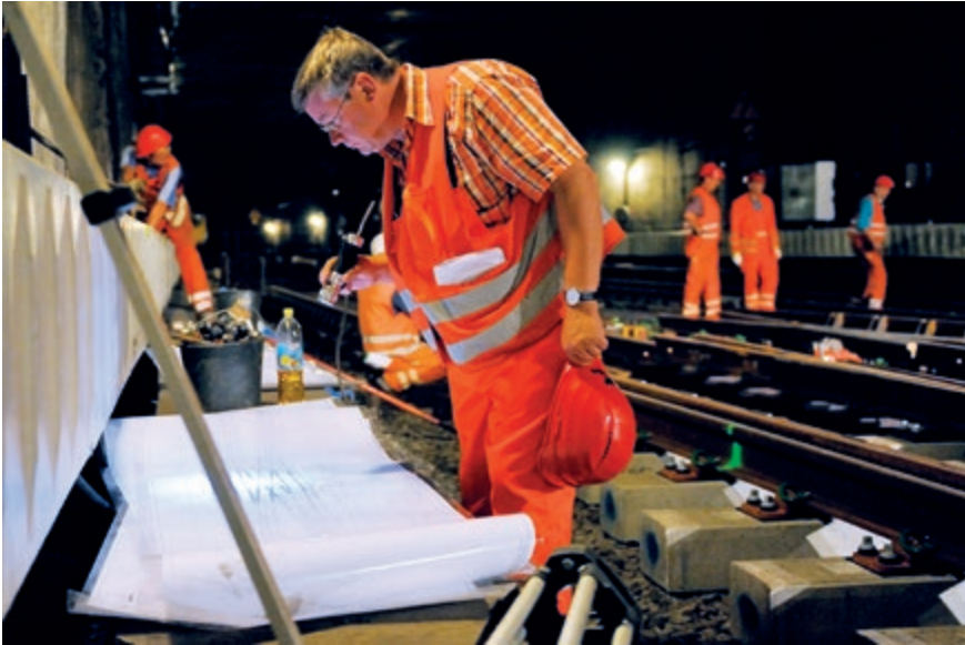
Tunnel work on the railway (Photo: Norwegian National Rail Administration)
