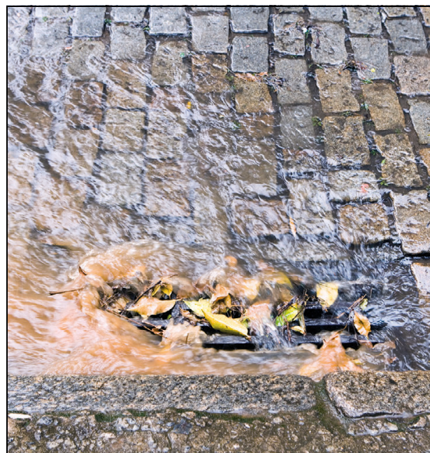
Figure 6.5 A street drain
