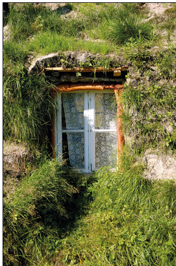
Figure 3.10 From a Sami settlement in Kaperdalen Museum, Troms, from the beginning of the 1900s. Window in a gamme (turf house) from the early 1900s, used by forest Sami until the 1960s.
