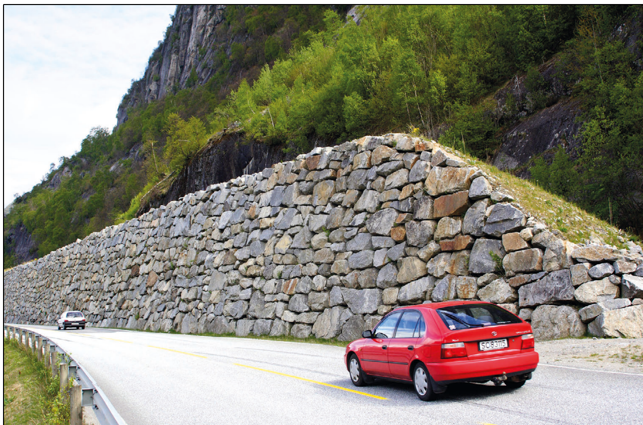
Figure 6.2 Rockfall barrier along a road
