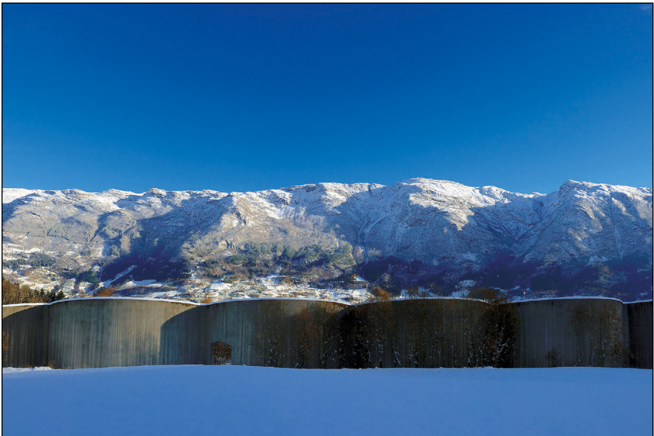
Figure 2.2 Concrete avalanche defence, Hardanger municipality
