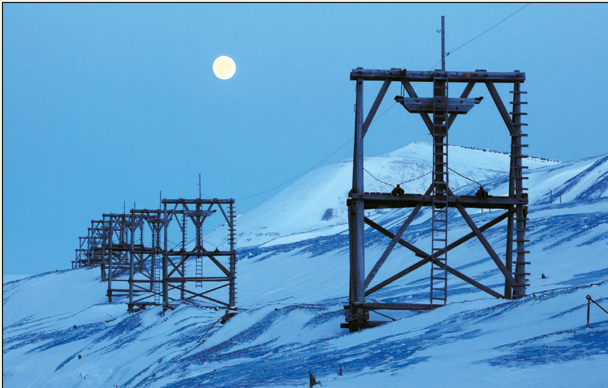
Figure 3.8 Supports for an aerial cableway from a coal mine in Svalbard, part of its protected cultural heritage.
