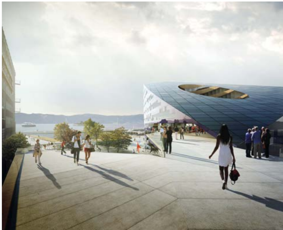
The sloping roof is covered with integrated photovoltaic panels. Ill.: Snøhetta/MIR
