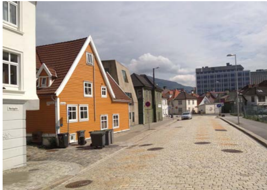
Façade toward the public area. Ill.: OPA Form Arkitekter
