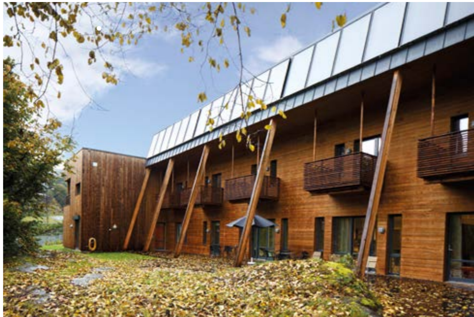
Façade toward the South, with solar thermal collectors. Photo: Vegard Giskehaug
