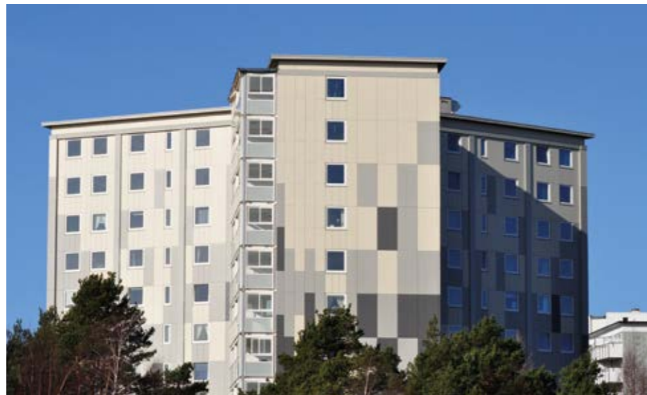
Apartment building upgraded March 2014. Photo: Svein Erik Bjorvand
