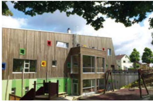
Façade toward outdoor area. Photo: ABACUS
