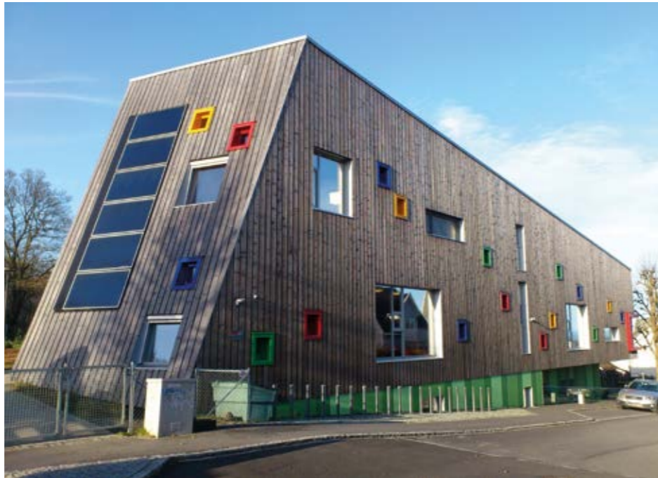
Southern façade with solar thermal collectors. Photo: ABACUS
