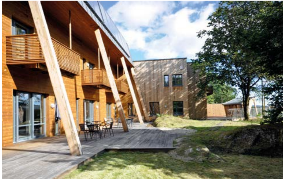
Façade toward the garden. Photo: Vegard Giskehaug
