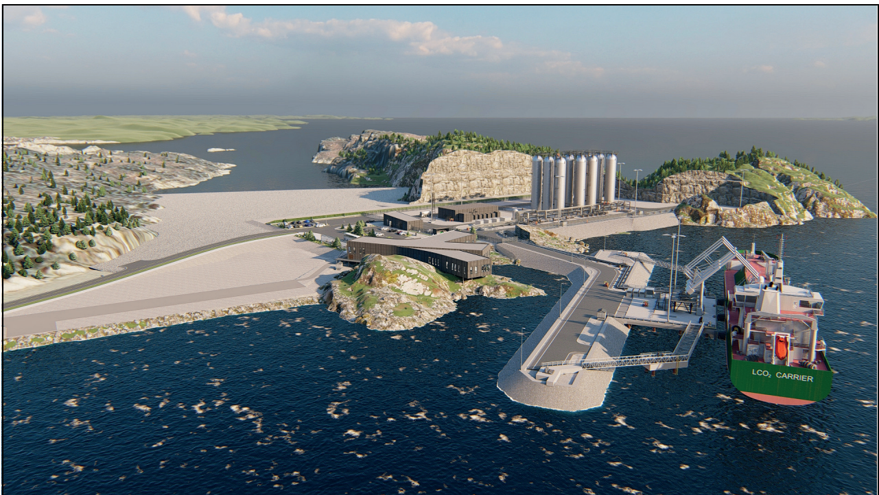
Figure 4.6 Illustration of Northern Lights' receiving terminal in Øygarden municipality
