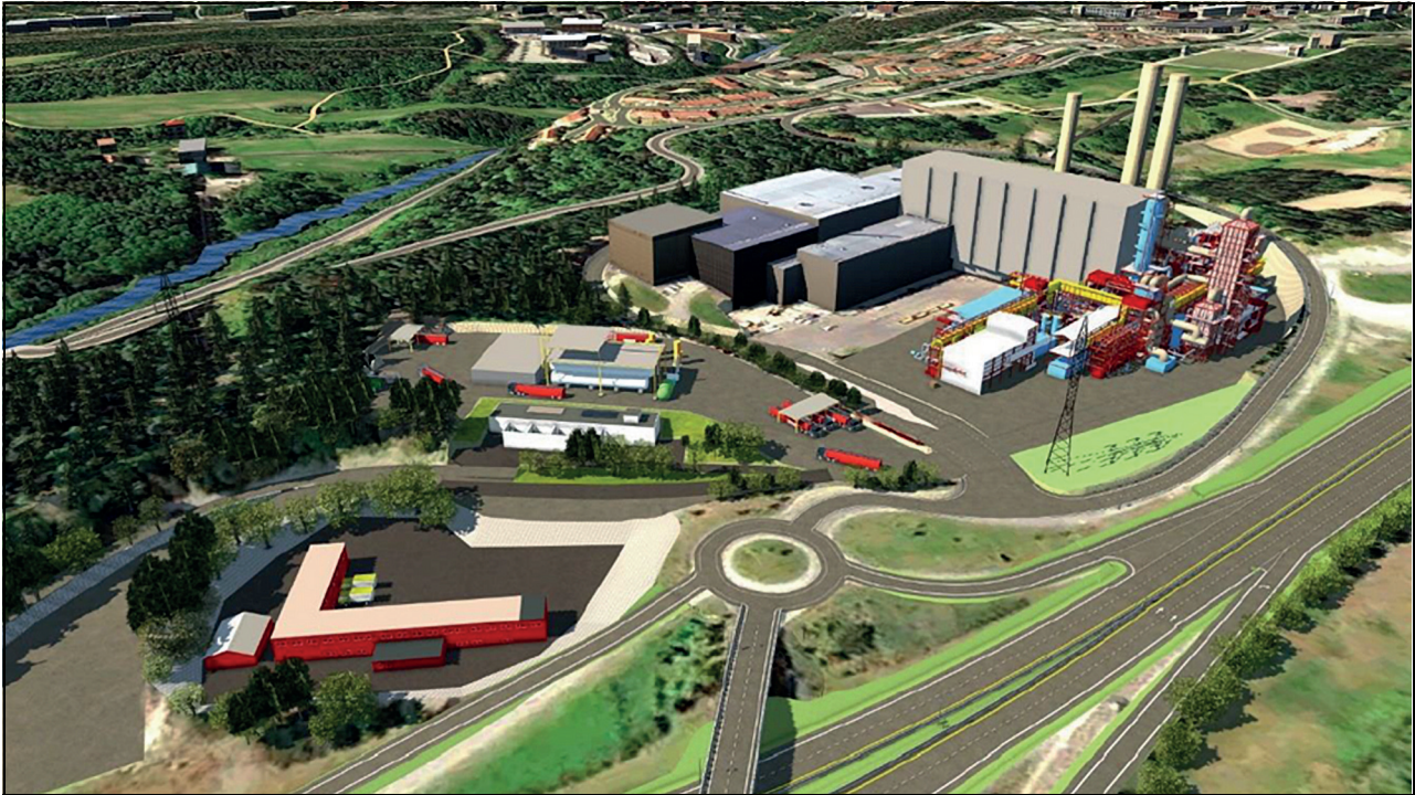
Figure 4.4 Fortum Oslo Varme's carbon capture facility
