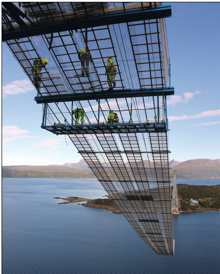
Figure 4.4 Hålogaland bridge under construction
