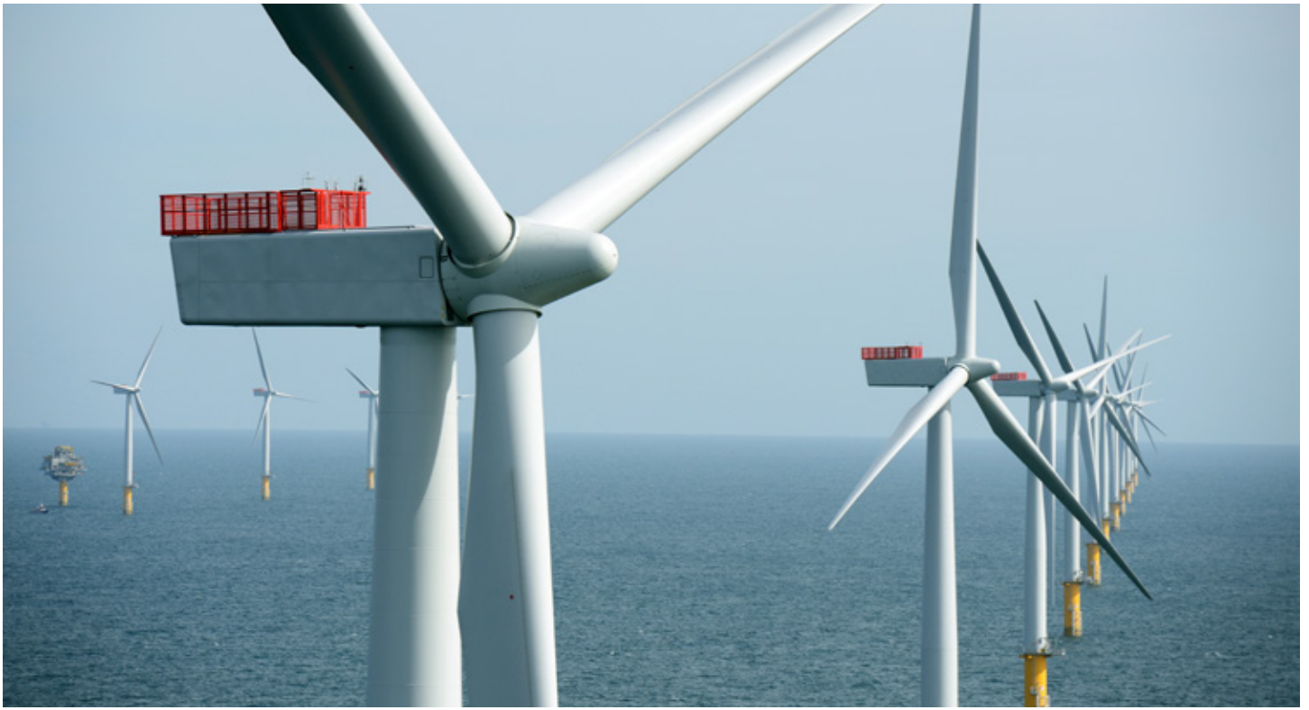
Offshore wind farm. Photo: Allan O'Neil/Equinor.
