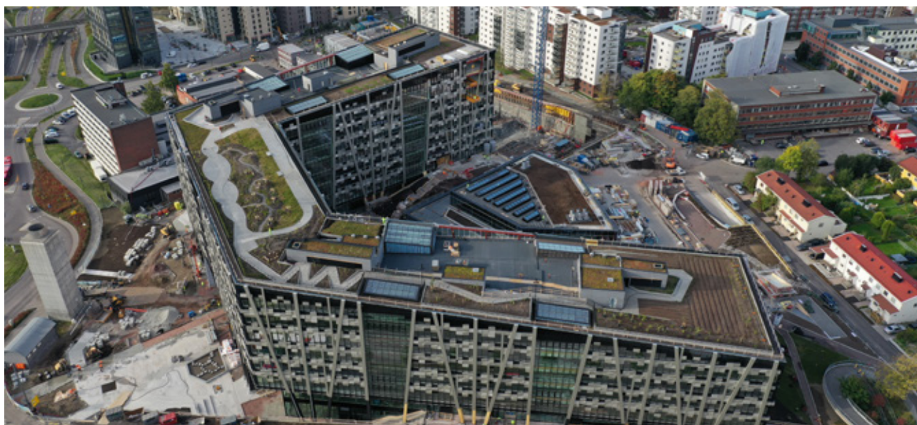
Økern Portal, Northern Europe's largest rooftop park covering 7,000 m 2 with allotments, beehives and recreation areas. Here, children and adults can learn about cultivation and circular systems. Waste from the building will be composted and used as fertiliser. Photo: Christian Grønvold Hansen.
