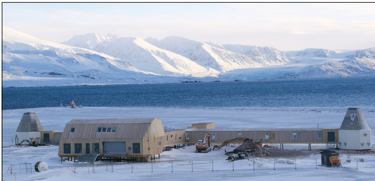
Figure 8.1 The Norwegian Mapping Authority's new geodetic observatory in Ny-Ålesund. The observatory is due to be completed in 2018.
